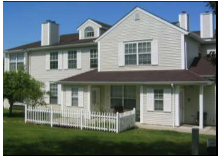
Grand Bay Apartments, Cleveland, Ohio
