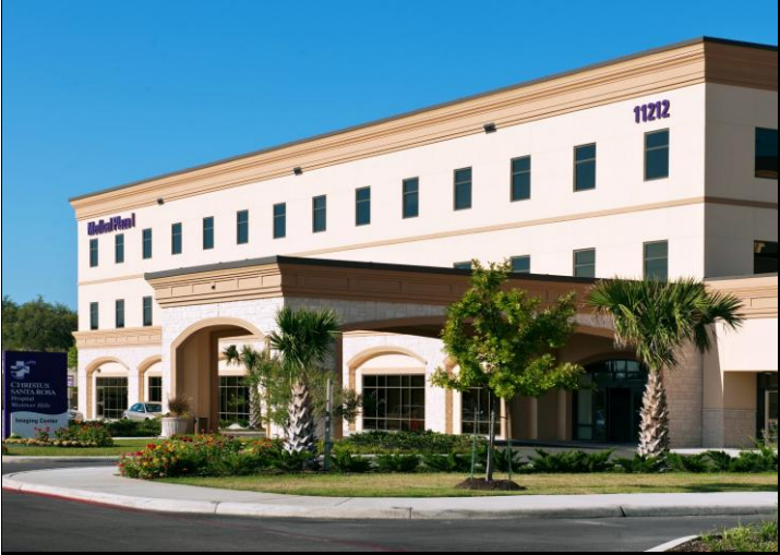
Christus Medical Office, San Antonio, TX
